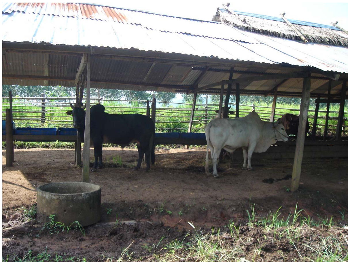
Cattle shed in Kanchanaburi, Thailand
